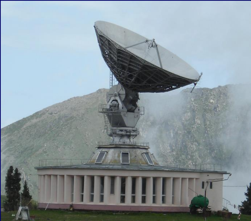
12 m parabolic dish Tian Shan mountains, 2735 m asl
